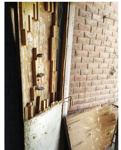
Conditions prior to renovation.
